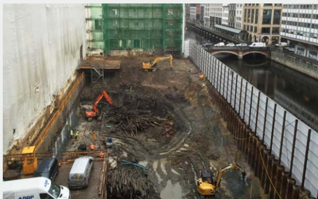
Demanding excavation at „Alter Wall“
